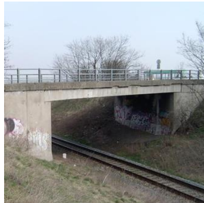
Figure 1. A side view of analyzed bridge
